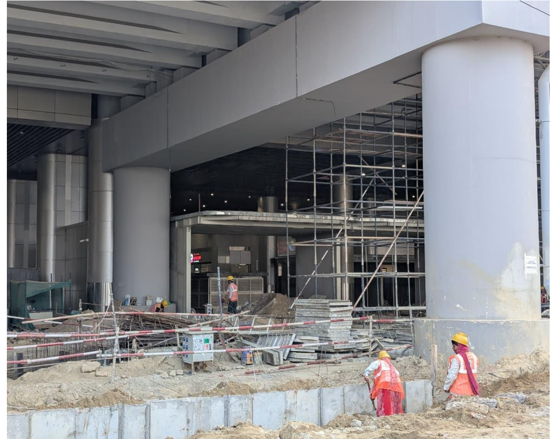
Glazing and terminal side columns, Services work ongoing.
