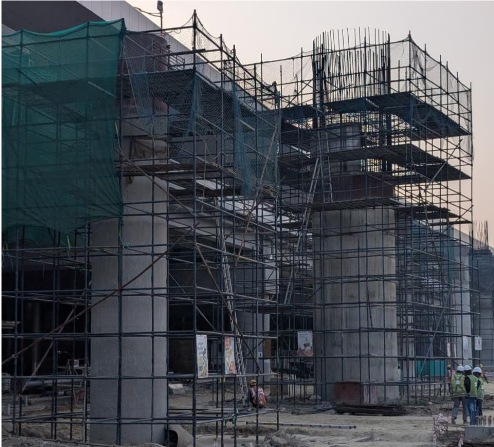
Phase 3 Canopy and Stack columns, construction ongoing. Structure work pending, Upon completion primary steel will be installed , MEP services will be completed which will make way for GFRP installation.
