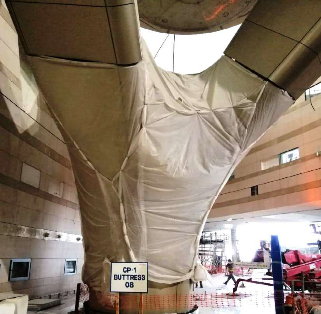
MTB CP1 BUTTRESS – ABU DHABI
